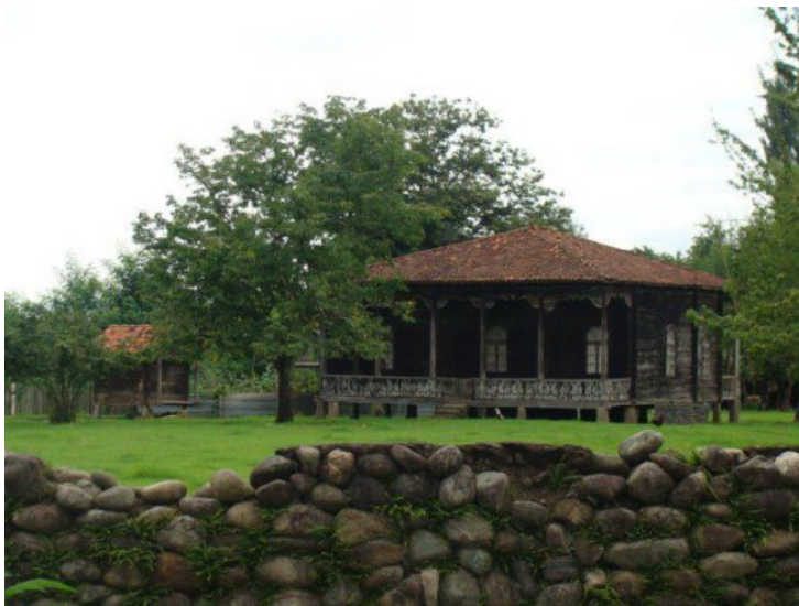
Figure 4.2. Oda: typical house in the western lowlands of Georgia. Made of chestnut timber. Roof formerly spruce or fir shingle, replaced with clay tiles. The house is based on stone supports to maintain a clearance from the soil and avoid dampness. Now the Museum of Shalva Radiani, a prominent literary critic of the 20th century. ( https://commons.wikimedia.org/w/index.php?curid=28830412 )
