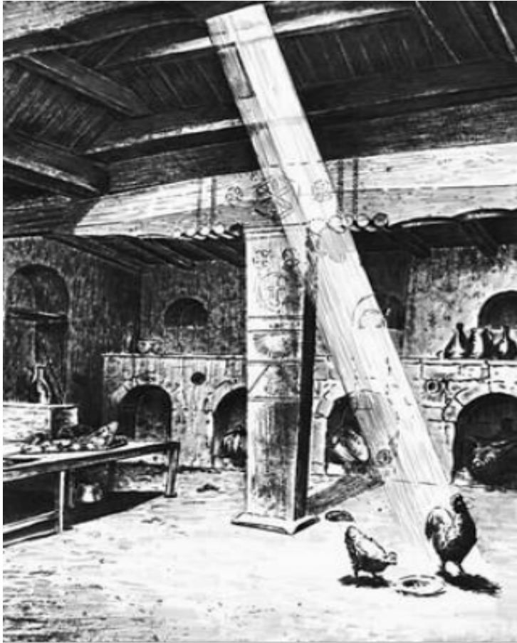
Figure 4.1. Darbazi: a typical house in the eastern lowlands of Georgia. Light comes from the window on the top of the roof. Dedabodzi (Mother Pillar) decorated with traditional symbols is in the centre to support the roof. ( http://bse.scilib.com/pictures/05/01/289985083.jpg ).
